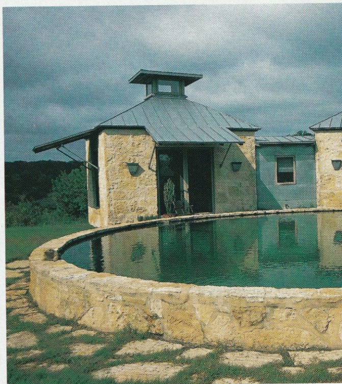
At Ramshead Ranch, San Antonio-based Lake-Flato Architects designed the house with its dramatic pools. This modern ranch house sticks close to tradition with the choice of building materials—buttery limestone and standing-seam metal roofs have adorned farm and ranch structures for more than 140 years. The round pool is actually a Texas-size pond for exotic koi fish.
